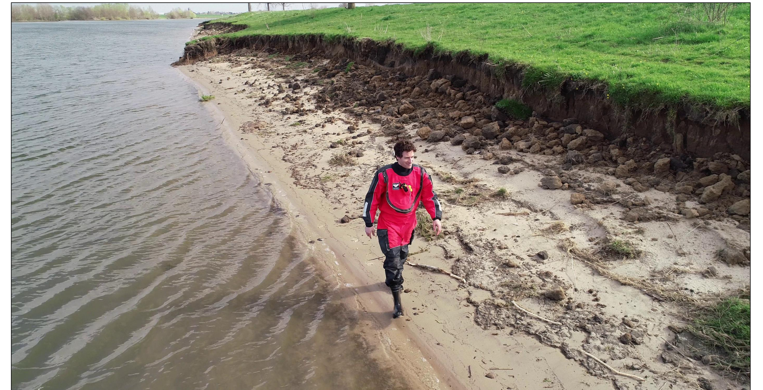
Inspection of eroding banks near Neerloon, the Meuse River.
