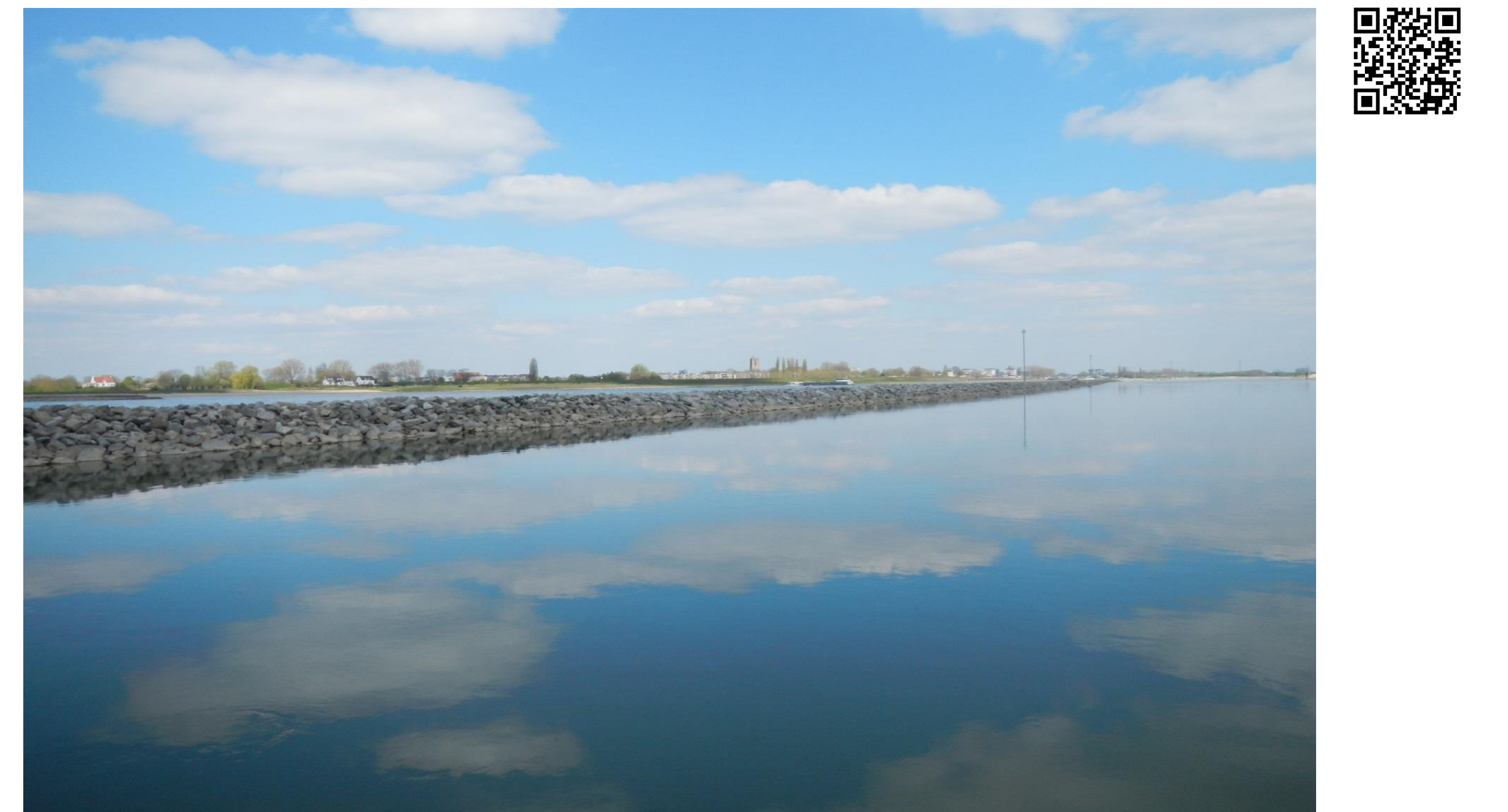
Figure 1: Photo of one of the longitudinal training dams constructed in the river Waal near the municipality of Dreumel
