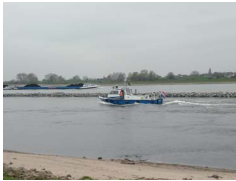
Figure 6. Longitudinal training dams (LTD pilot).
