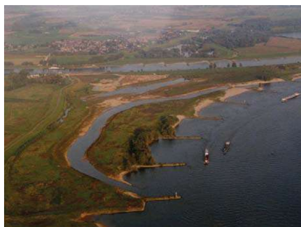
Figure 1. An example of a nature rehabilitation project along the Waal River (The floodplain Klompenwaard). Excavation of the top clay layer of the floodplain and a secondary channel will create more room for hydro-morphodynamics and suitable conditions for riparian biodiversity.
