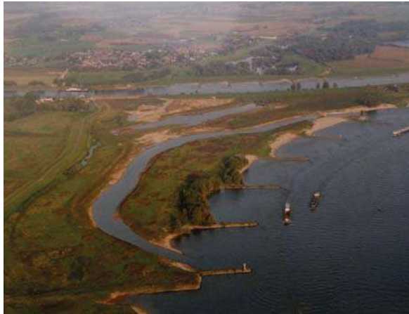
Figure 4. An example of a nature rehabilitation project in the floodplain Klompenwaard along the river Waal in the Netherlands (From Smits et al. , 2003). Excavation of the top clay layer of the floodplain and a secondary channel will create more room for hydro-morphodynamics and suitable conditions for riparian biodiversity.
