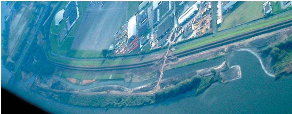
Figure 1. The construction of a meandering side channel along the river Bergsche Maas at Dombosch, near Geertruidenberg (The Netherlands).
