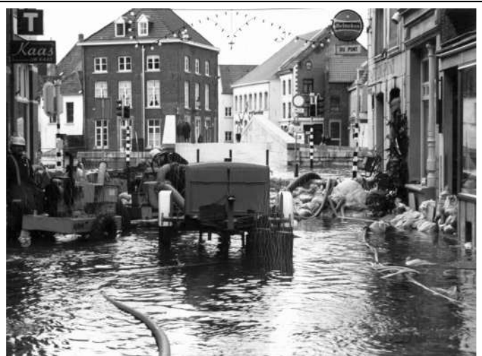
Figure 1. Flooding in the city of Roermond, 1995.
