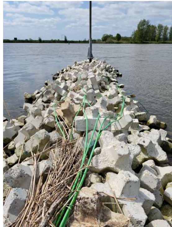
Figure 1: Photograph of the extended flexible groyne in the IJssel river (source: Robert Groenewege)
