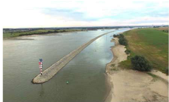
Figure 1: Longitudinal training dam in the Waal River near city Tiel (photo F. Collas, Radboud University Nijmegen)
